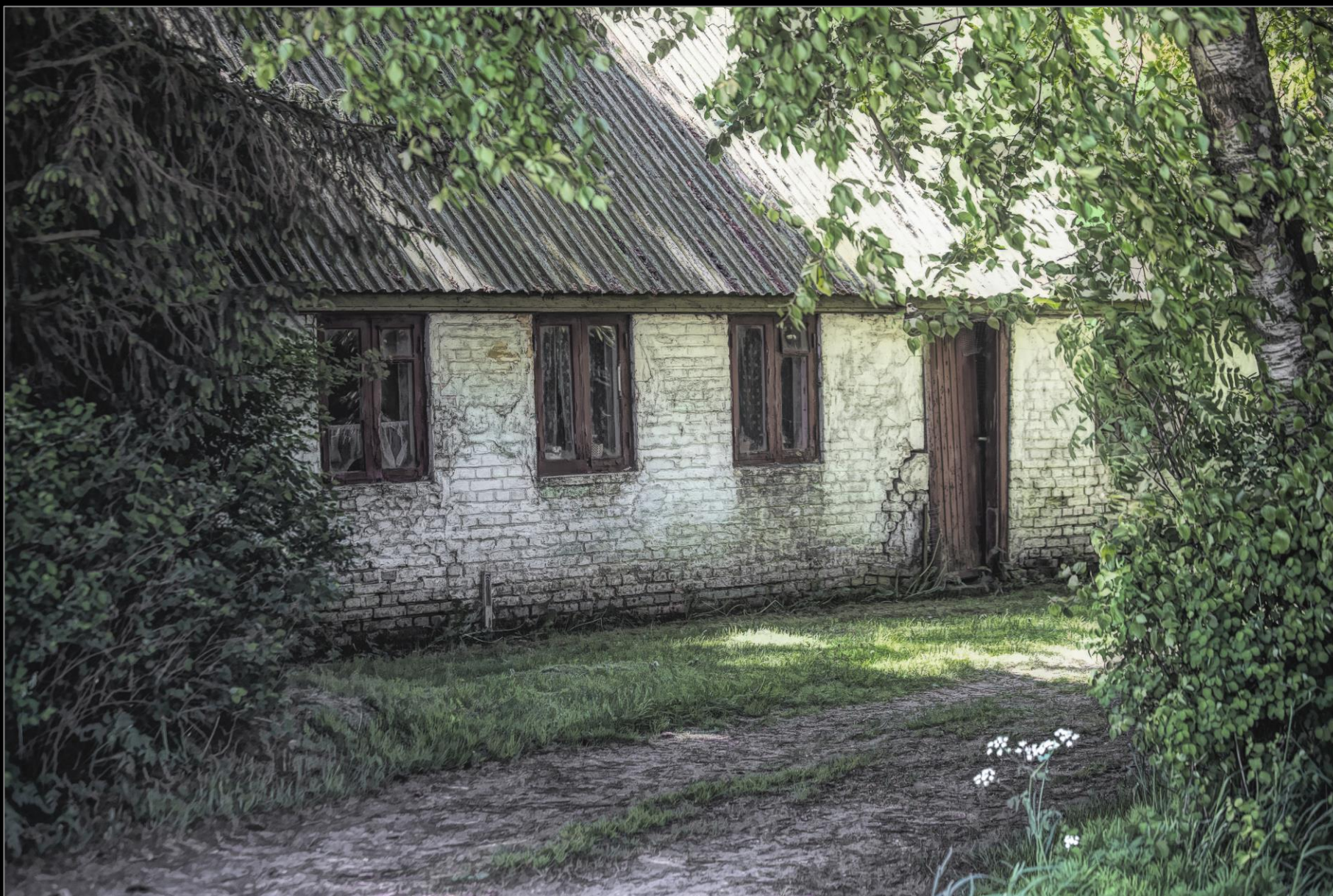
A house south of the village Øster Hurup, August 2018
