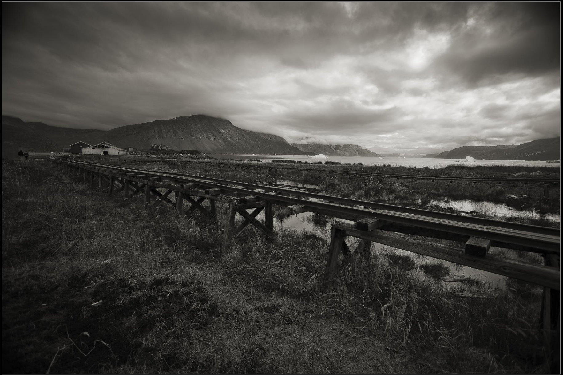
The track for transporting of cod, Qornoq, July 2010
